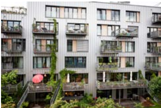
2008–2013, Completed | designed by stekke + fraas | commissioned by brutopia asbl
